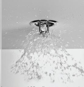
Water flowing from a sprinkler head can exceed 25 gallons per minute!
